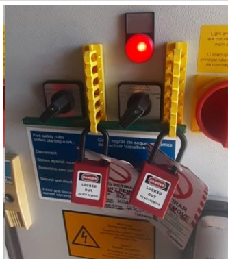
Barra horizontal fijada sobre los sopores ya instalados. Dicha barra impide el giro de los dos selectores. Horizontal bar fixed on the supports already installed. This bar prevents the two selectors from turning.
