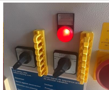
Soportes adhesivos pre-instalados sobre el frontal del armario Adhesive brackets pre-installed on the front of the cabinet.
